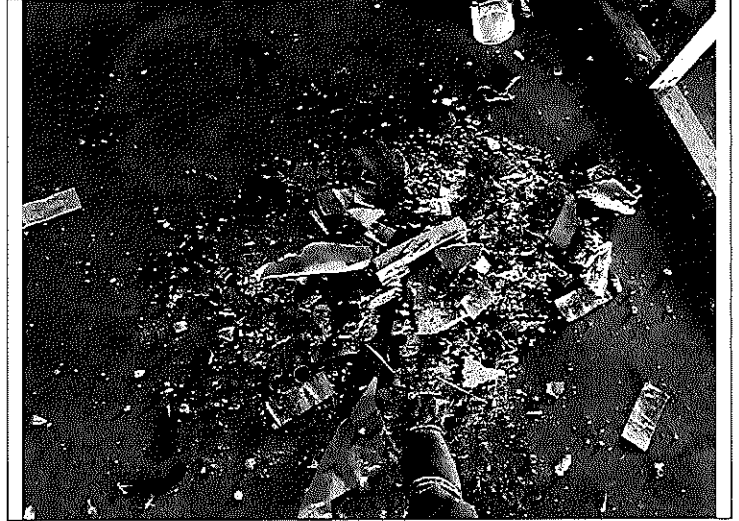
10. View of the ACM construction debris located on the floor inside Building A.
